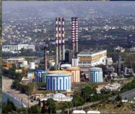
Thermoelectric power plant
