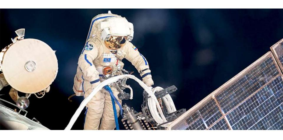
Installation of an antenna for the ICARUS system at the International Space Station ISS
